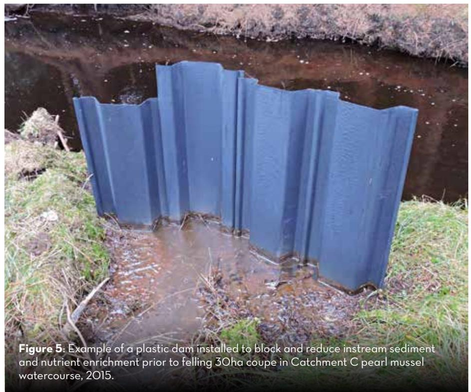
**Figure 5:** Example of a plastic dam installed to block and reduce instream sediment and nutrient enrichment prior to felling 30ha coupe in Catchment C pearl mussel watercourse, 2015.
